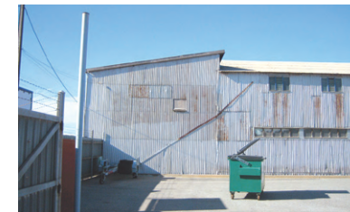
Figure 3.50 North west corner of Shed F indicating an addition to the north.
