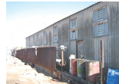
Figure 3.51 East boundary wall of Searles. Asbestos cladding evident
