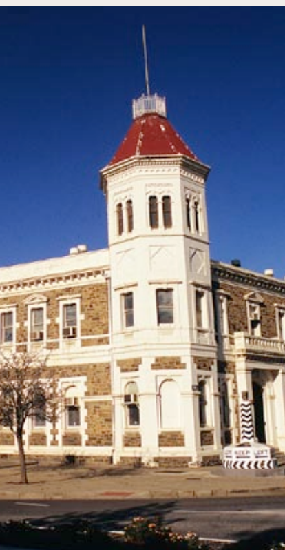
Above: The Customs House, Port Adelaide, is deteriorating rapidly through neglect.
