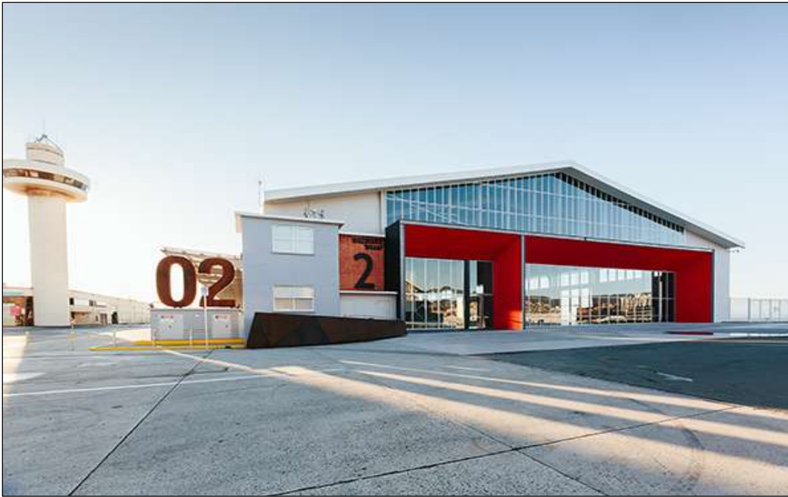
Figure 6: Macquarie Wharf No. 2 Cruise Terminal is one of Hobart's newest waterfront event spaces catering for medium to large scale corporate functions, events, concerts and expos (photo TasPorts)
